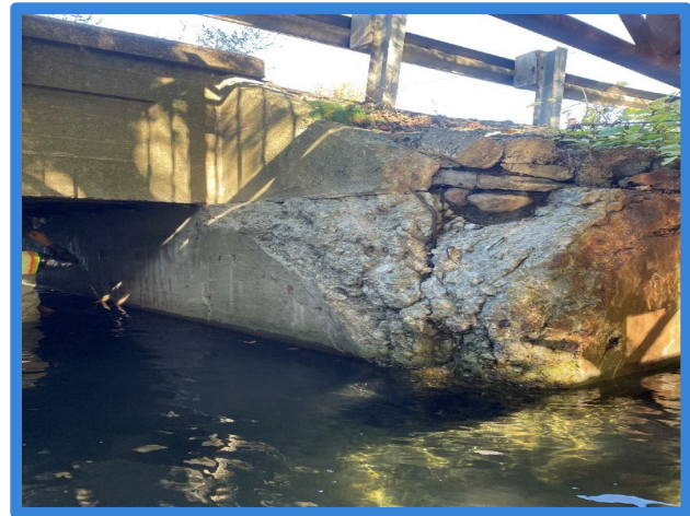
Austin Lake Drain Culvert Deteriorated Spillways
