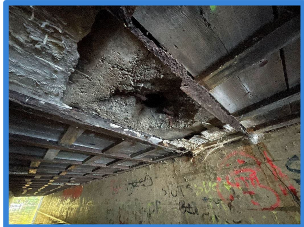
Portage Road Culvert Failed Beams
